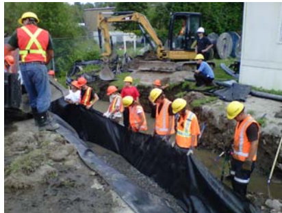
Group effort in preparing footings for new culvert
